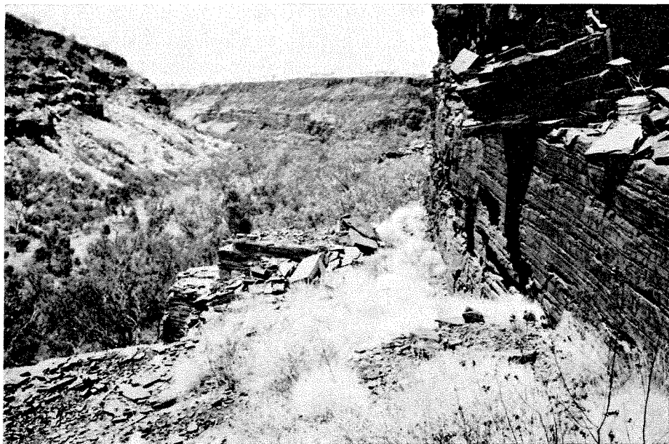
Figure 68. Abandoned surface bench working of crocidolite on the north side of Snell Gorge (Plate 8). The steep gorge sides severely limit the mineable bench width. The view is in a southwesterly direction with the western side of Yampire Gorge in the distance.
