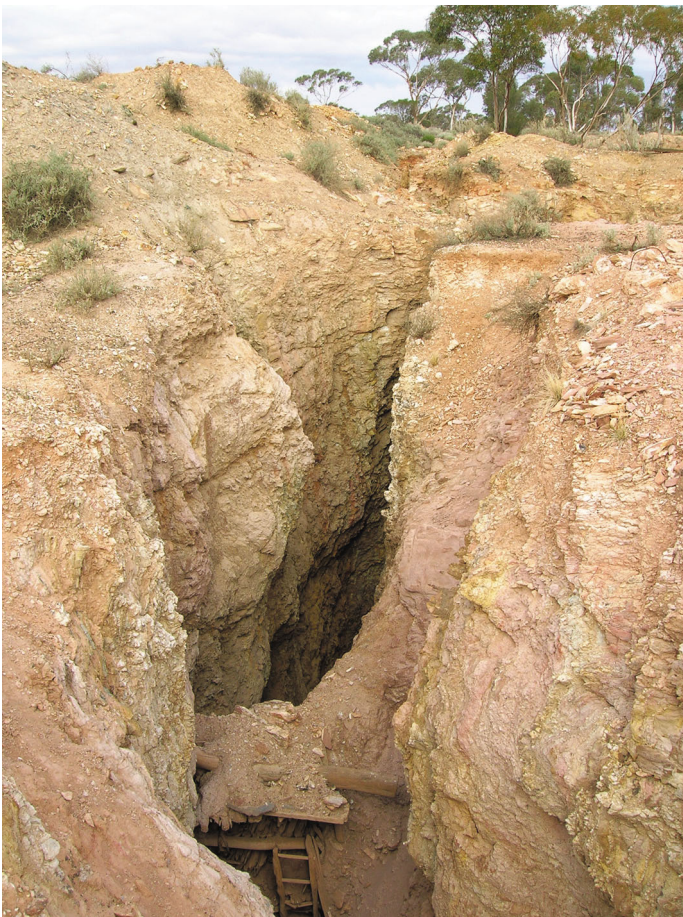
Collapsing partially banded, vertical 10 x 6 m open stope at the Duke mine site, 3.1 km northwest of Broad Arrow. This deep (5–10 m) multi-level development contains remnants of stope timbers and ladder-ways.
