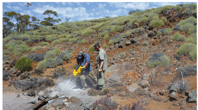
Drilling granite in the Albany Fraser Orogen to recover samples for Hf isotopic analysis
