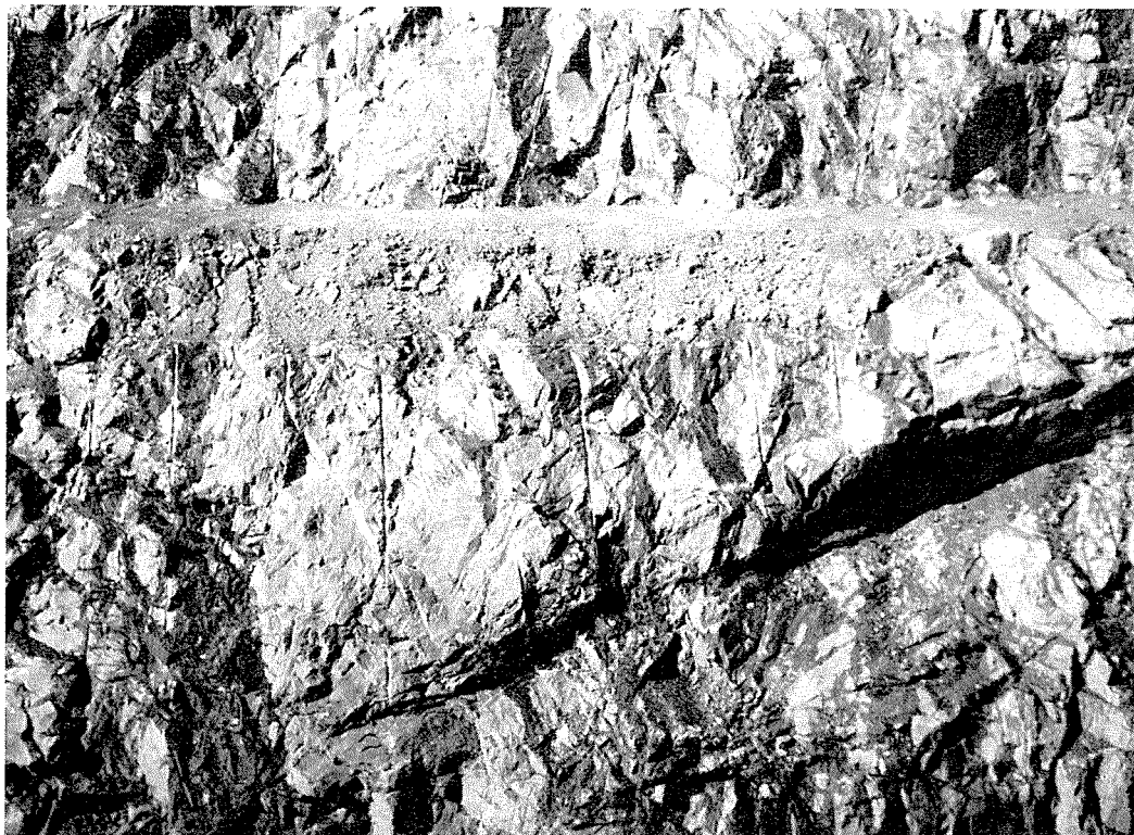
A. A steeply dipping joint plane has caused overbreak at the toe of a batter. Note also the loss of the berm edge, now filled with rubble, because of numerous blasting cycles; FN 1241.
