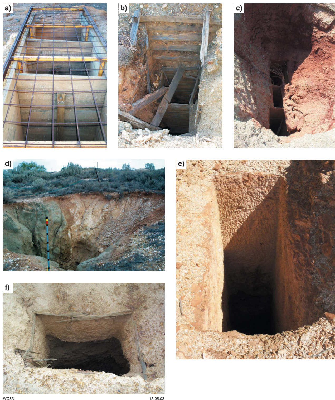
Figure 63. Various types of shafts and their dimensions (length \times width, and depth): a) three-chambered shaft (3.5 \times 1.2 m, >10 m deep) with collar timbers in good condition (1 km northwest of Bardoc; Zone 51, MGA 335217E 6642975N); b) two-chambered shaft (2.6 \times 1.5 m, >10 m deep) with collar timbers in poor condition, resulting in collapse of the upper shaft collar (5.5 km north of Coolgardie; Zone 51, MGA 323893E 6579364N); c) three-chambered shaft (4 \times 1.2 m, >10 m deep) with severe subsidence of the upper shaft collar caused by shaft collar collapse in unstable near-surface conditions (2.5 km north of Kanowna; Zone 51, MGA 365864E 6615065N); d) 10 to 20 m-deep shaft with severe collar collapse, and a subsidence cone that is encroaching on the surrounding, three-strand wire fence in poor condition (1 km northeast of Coolgardie; Zone 51, MGA 325280E 6574870N); e) competent shaft collar (1.8 \times 0.7 m) in firm saprolite after porphyry (10 km southwest of Coolgardie; Zone 51, MGA 319335E 666110N); f) shaft collar (1.2 \times 0.7 m) showing undercutting beneath hard caprock and remnant collar timbers in poor condition (6 km northwest of Bardoc; Zone 51, MGA 331892E 6646764N)
