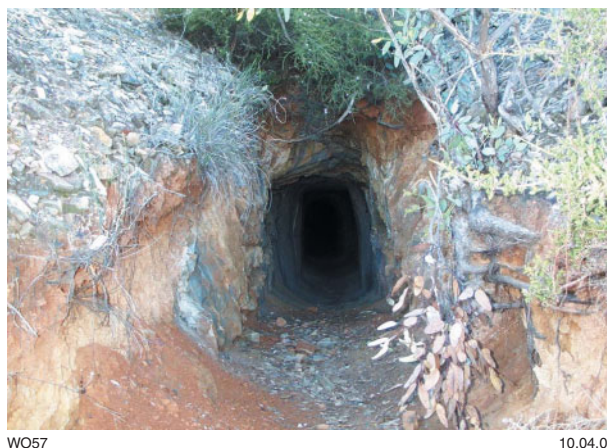
Figure 28. Adit of 1.5 m height and 1 m width (9 km east of Ravensthorpe; Zone 51, MGA 235048E 6277910N)
