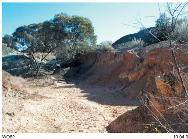
Figure 38. Typical shallow pit/quarry, 40 m long, 10 m wide, and 2.6 m deep (6.5 km northeast of Coolgardie; Zone 51, MGA 329220E 6579005N)
