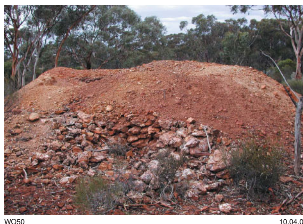
Figure 16. Typical shaft with a full bund, between 1 and 3 m high (13.5 km east of Boulder; Zone 51, MGA 369080E 6592470N)
