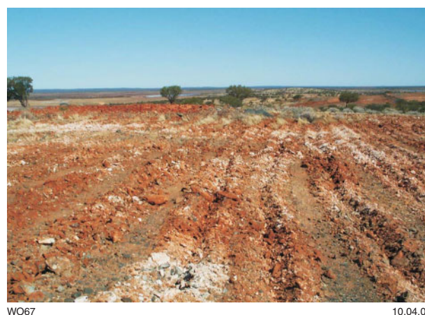
Figure 49. Typical rehabilitated area showing ripped ground over workings (34 km north of Leinster; Zone 51, MGA 259148E 6940971N)
