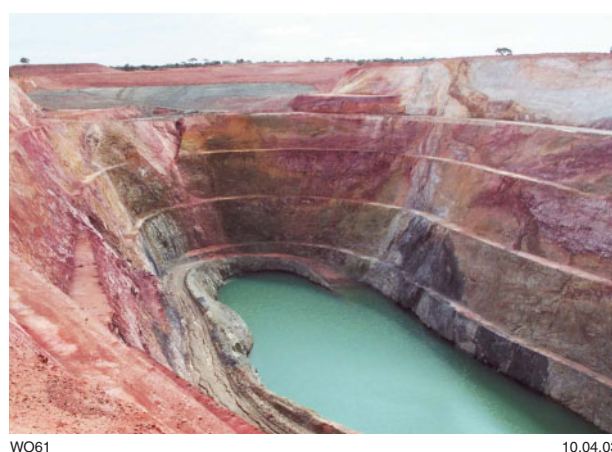
Figure 36. Typical deep pit/quarry, 300 m long, 180 m wide, and more than 20 m deep, with a limited access ramp (1.5 km south of Broad Arrow; Zone 51, MGA 339482E 6629793N)
