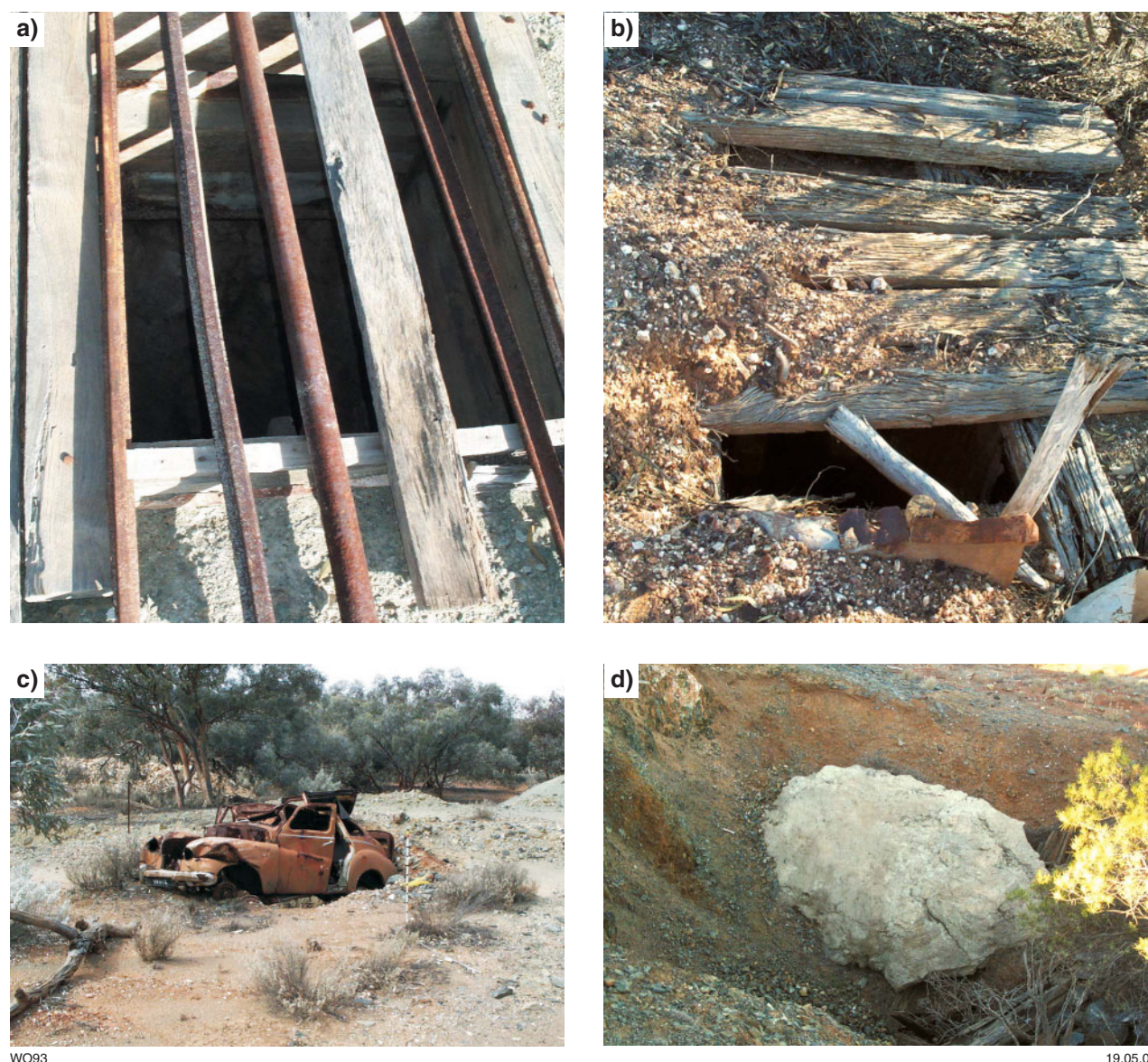
Figure 65. Various types of seals: a) partial seal of loose timber and steel rails has improved the visibility of this shaft ( 1.3 \times 1.3 m, >10 m deep), but may not prevent accidental entry (6 km northeast of Coolgardie; Zone 51, MGA 328239E 6579062N); b) partial seal of loose timber partially conceals this shaft ( 1.5 \times 1 m, 5–10 m deep; 10 km southwest of Coolgardie; Zone 51, MGA 319700E 6565450N); c) car disguises a shaft ( 3 \times 3 m, 5–10 m deep), but may not protect from accidental entry (3.5 km northeast of Coolgardie; Zone 51, MGA 327140E 6576810N); d) apparently inverted concrete seal in a collapsed underground working, now 5 \times 5 m, and 2–5 m deep (8 km south of Coolgardie; Zone 51, MGA 322709E 6566601N)
