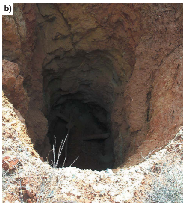
Figure 68. a) Subsidence of an abandoned working (4 × 3 m, 5–10 m deep) adjacent to the road as shown in Figure 67 (8 km south of Coolgardie; Zone 51, MGA 322782E 6566561N); b) downhole view of the subsidence shown in (a)
