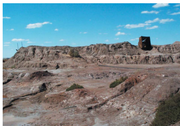
Figure 54. Typical tailings dump, 160 m long, 75 m wide, and 3 m high (6 km southeast of Boulder; Zone 51, MGA 360054E 6589865N)
