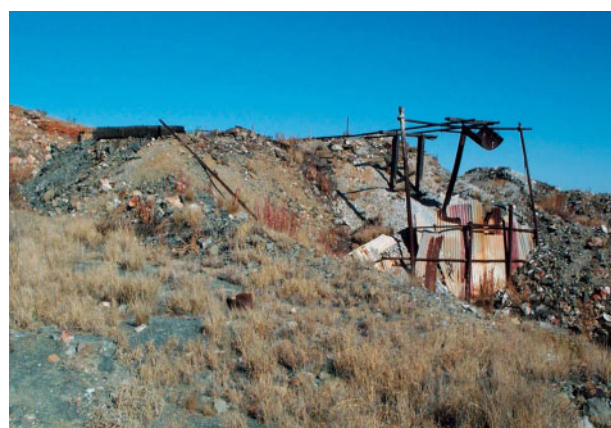
Figure 57. Ramp/tramway, 30 m long, 15 m wide, and 4 m high (35 km south-southwest of Meekatharra; Zone 50, MGA 633774E 7025299N)
