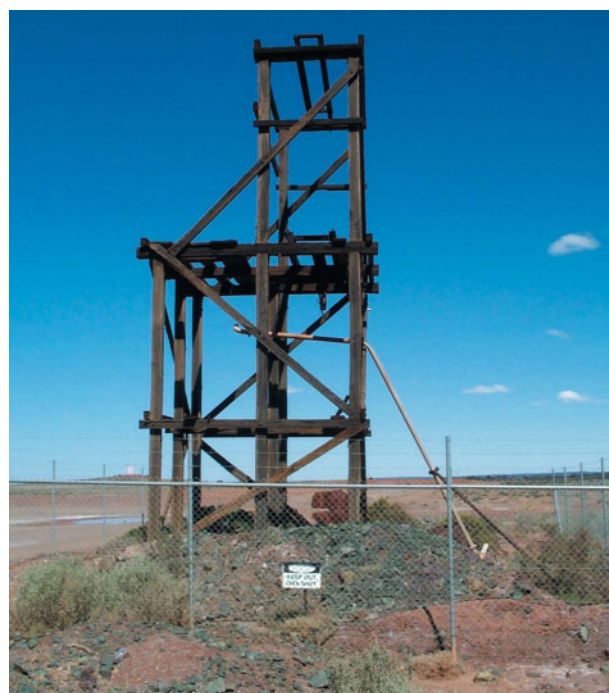
Figure 61. Nine-posted headframe and stand, 3 m long, 3 m wide, and 8 m high (3 km southeast of Boulder; Zone 51, MGA 357738E 6591584N)
