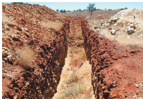
Figure 40. Typical mechanically (excavator or backhoe) excavated costean/trench, 30 m long, 2 m wide, and 0–5 m deep, with a partial bund to 2.5 m height (35 km south-southwest of Meekatharra; Zone 50, MGA 633436E 7025882N)
