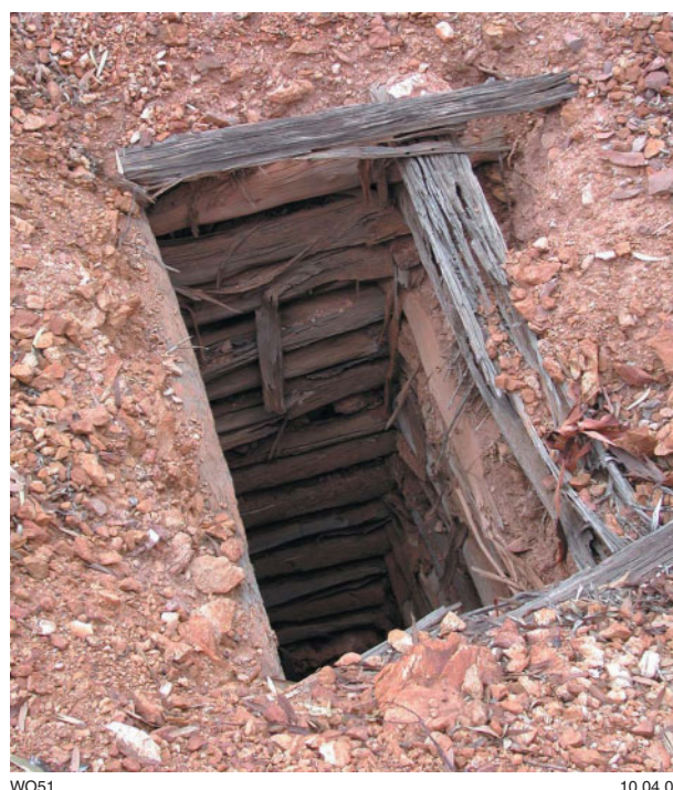
Figure 17. Timbered collar of the shaft shown in Figure 16. Shaft is 2.2 m long, 1 m wide, and 5–10 m deep
