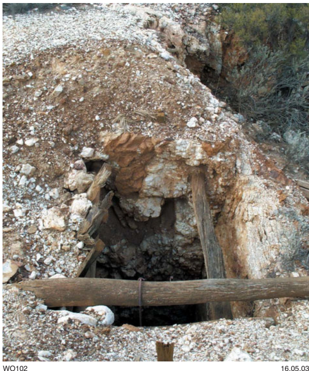
Figure 70. Shaft (2 × 1.5 m, 10–20 m deep) on a sheared contact (290° strike and 80°N dip) of a highly fractured and folded quartz vein (2 km northeast of Coolgardie; Zone 51, MGA 326060E 6575260N)
