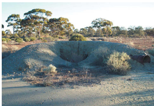
Figure 19. Typical shaft with a partial bund up to 1.1 m high. The shaft is 1.4 m long, 1 m wide, and 5–10 m deep (9 km northwest of Bardoc; Zone 51, MGA 330813E 6649318N)
