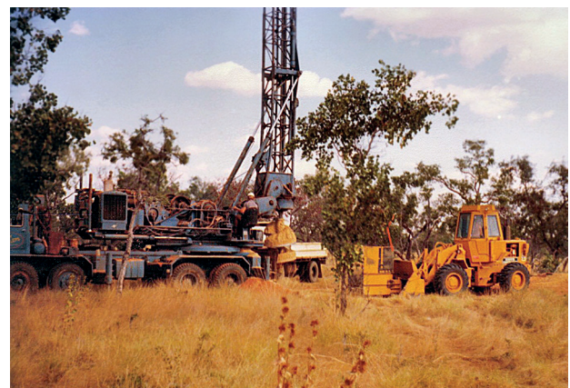
Figure 7. Hughes auger undertaking scout bulk sampling (photo by G Boxer, 1979)
