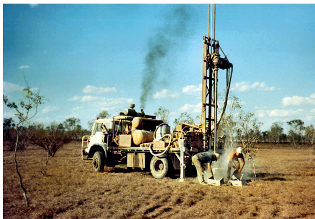
Figure 5. Exploration RAB drilling (photo by G Boxer, 1979)
