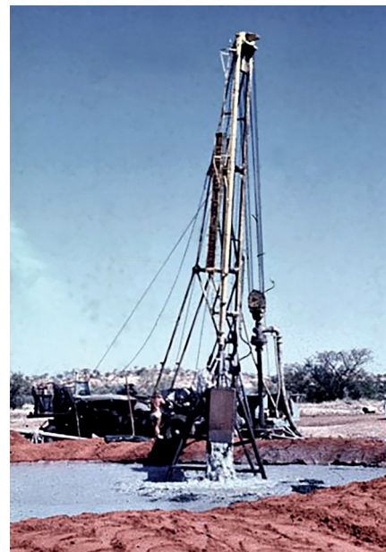
Figure 6. Wirth large-diameter drill sampling (photo by CB Smith, 1979)
