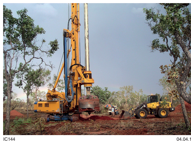
Figure 43. Bauer BG36 rig in action on the E4 J-channel (photo by GMI Rockett)
