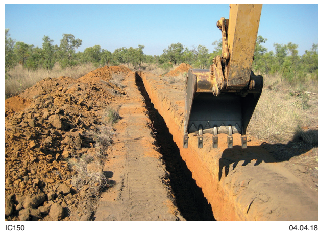
Figure 49. Trench sampling downstream on the E9 North western channel (photo by GMI Rockett)
