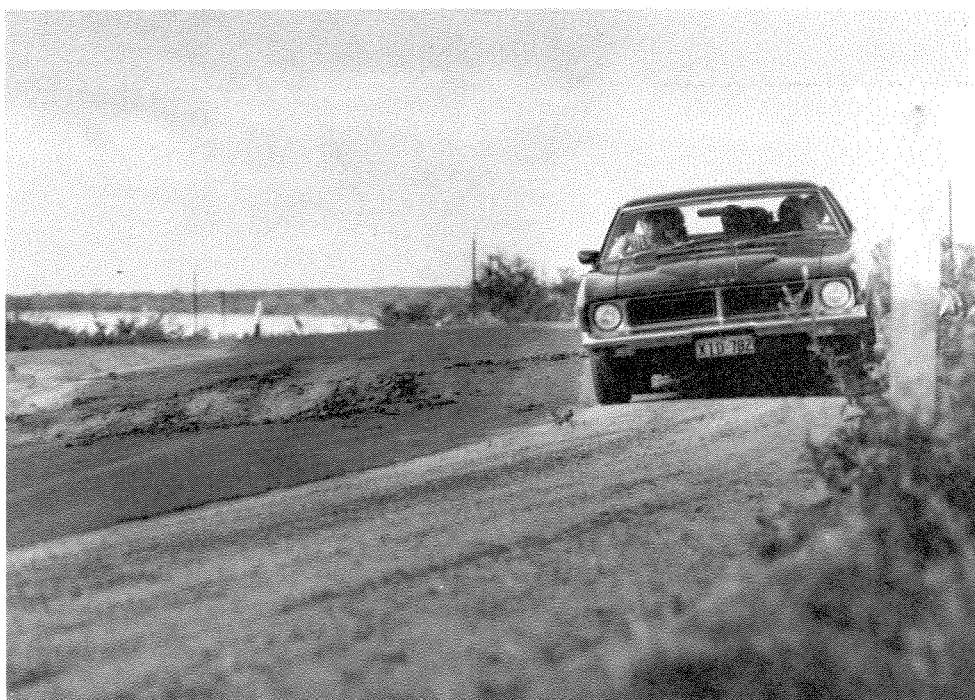
Figure 41. Road damage at the scarp of the Cumming Fault (photo: W.A. Newspapers) (GSWA 18774)
