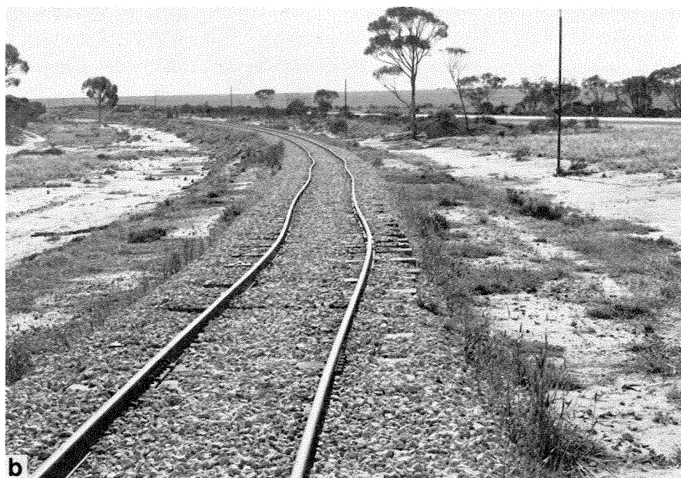
Figure 42. Damage to the railway line north of Cadoux: (a) vertical and left-lateral displacement at the Kalajzic Fault, (b) compressional damage about 1.3 km north of Cadoux (GSWA 18775)
