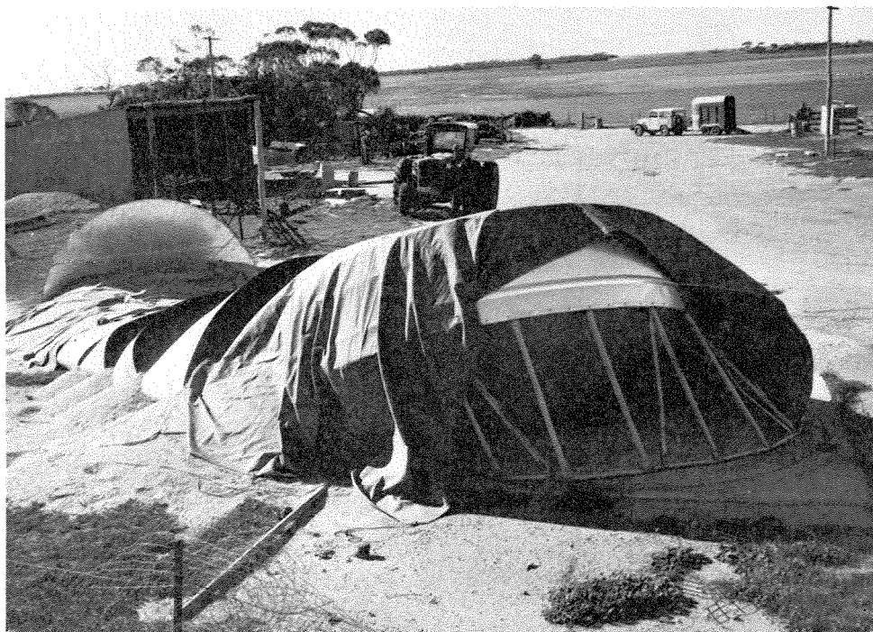
Figure 44. The collapse of a wheat silo on the Robb property: the silo has fallen to the northeast ( 047^{\circ} ) while the base has moved north ( 001^{\circ} ) (GSWA 18777)
