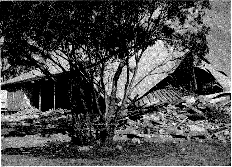
Figure 29. Cadoux Town Hall: the western wall and the block wall on the northern side have suffered total collapse. The frame structure at the rear of the building remains intact (GSWA 18762)
