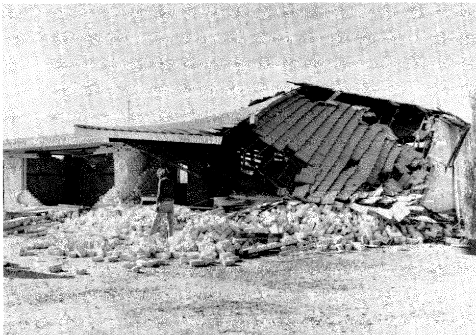
Figure 30. Cadoux Masonic Lodge: the western walls collapsed westward causing partial collapse of the roof (photo: W.A. Newspapers) (GSA 18763)
