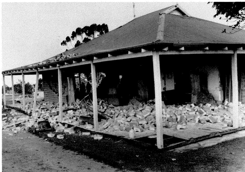
Figure 34. Damage to the house of Mr. E.W. Cumming: brickwork has collapsed while the timber-framed verandah and roof have remained intact (photo: W.A. Newspapers) (GSA 18767)
