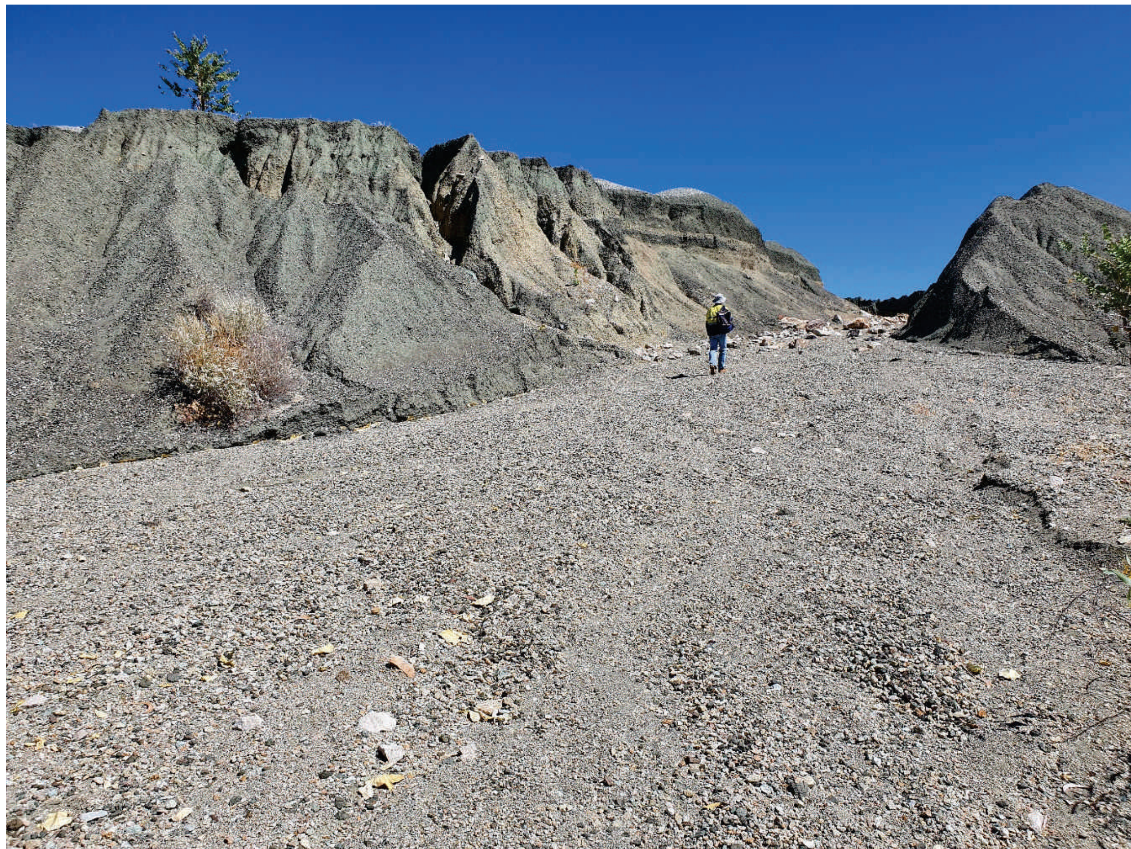
E4 Lights Stockpile erosion blowout and sediment fan
