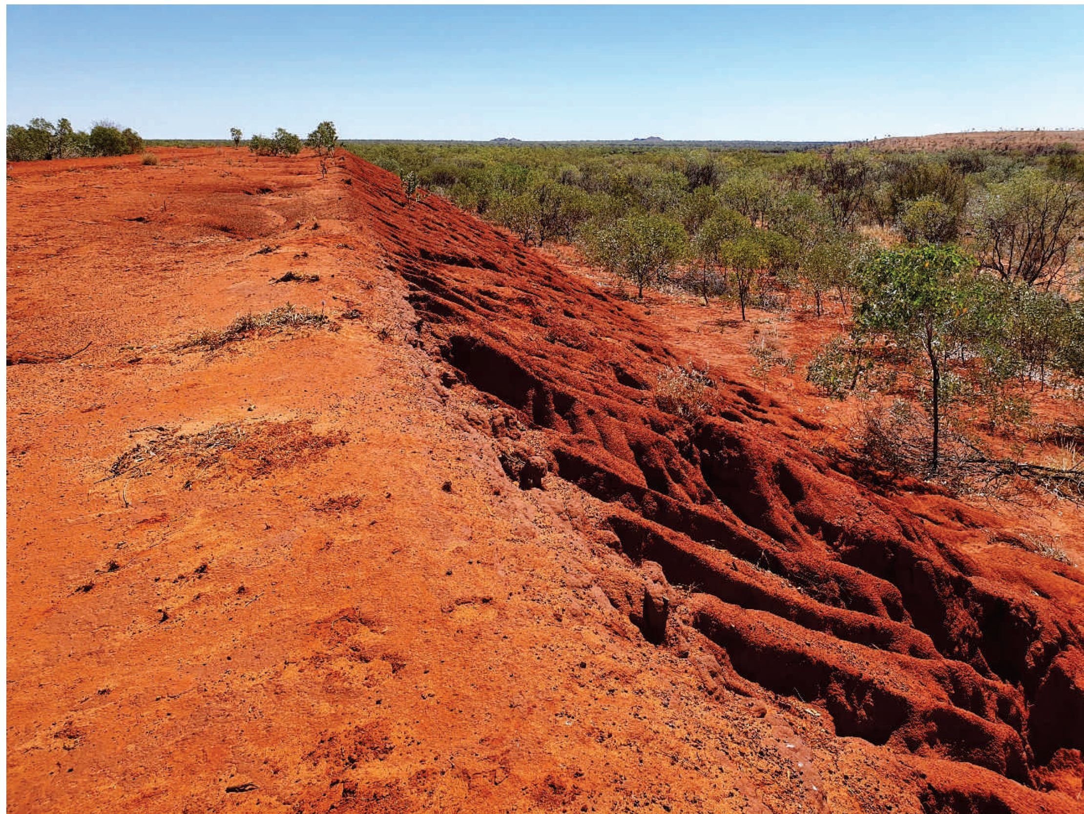
E4 TSF 2A northwestern wall showing significant surface erosion, gullying and tunnelling
