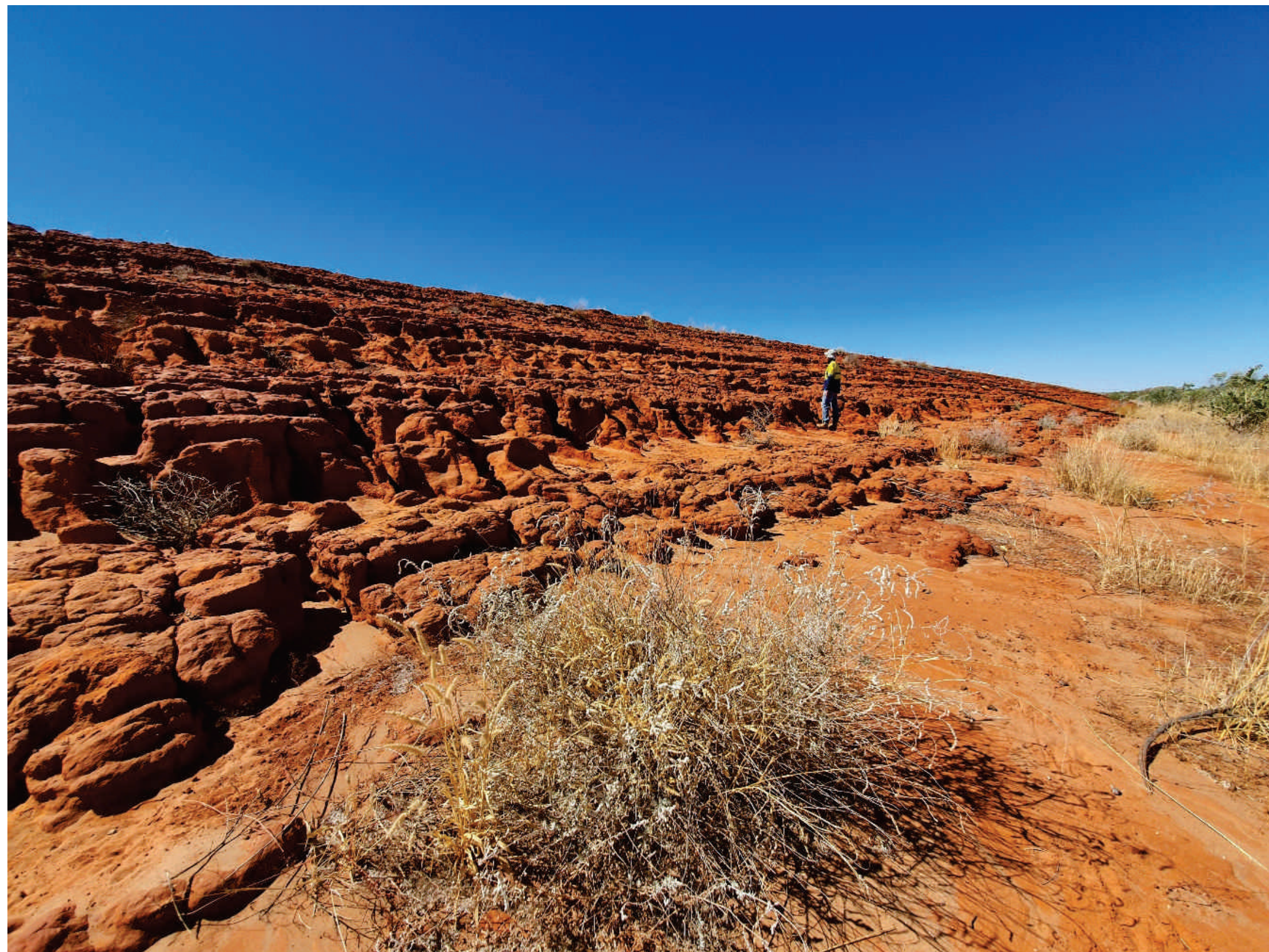
E9 TSF 1D significant gully erosion on the western wall of Cell 3
