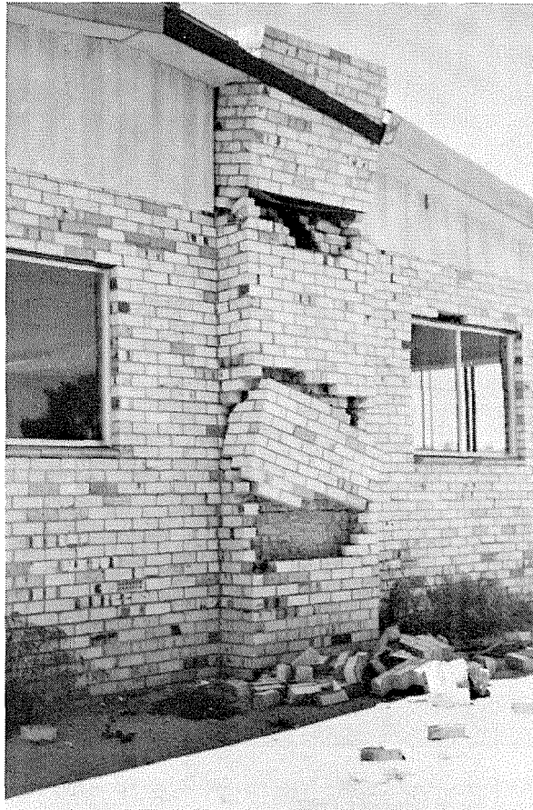
8. Chimney of the Meckering Golf Club house, damaged by the main earthquake and progressively wrecked by aftershocks.
