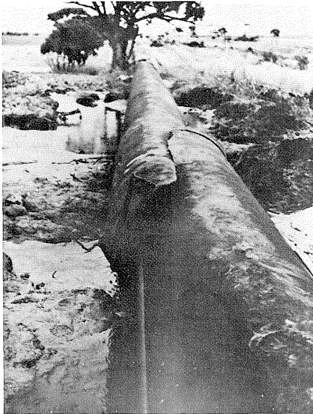
9. Impaction of the Goldfields Water Supply 76cm pipeline at the Meckering Fault, 4km southwest of the town. The compression at this point was 1.32m.
