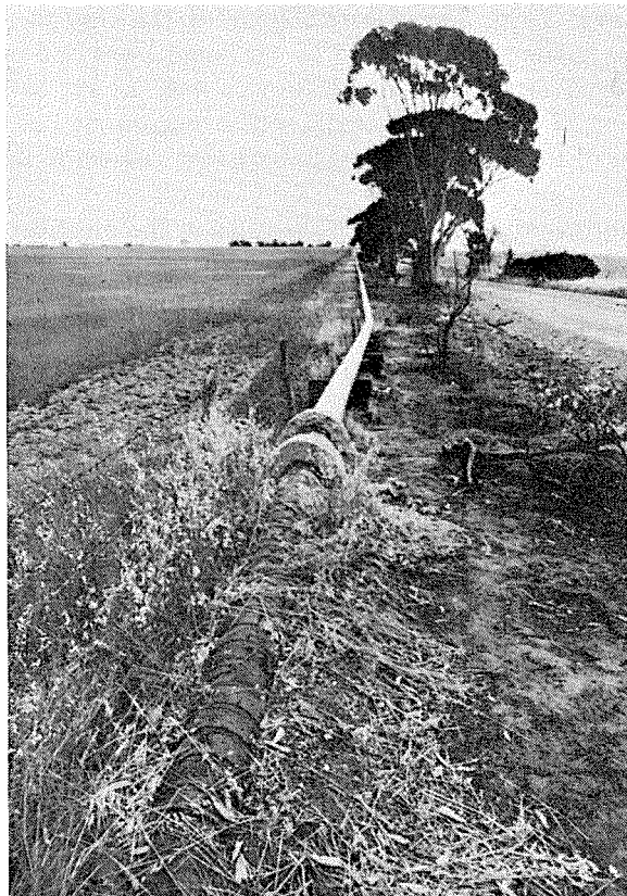
10. The Meckering-Goomalling pipeline at the Meckering Fault, 1.6 km northwest of the town. The original line of the pipe can be seen from the position of the abandoned pipe support.
