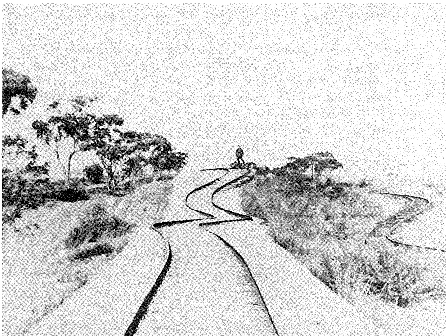
11. Distortion of the standard and narrow gauge railtracks at the Meckering Fault. The figure is standing on the 3 m-high fault scarp.
