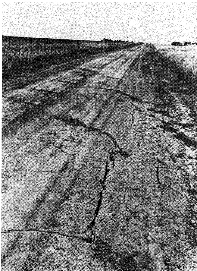
59. The Backscarp Zone: minor faulting on road 12865, 14 km south-southeast of Meckering.
