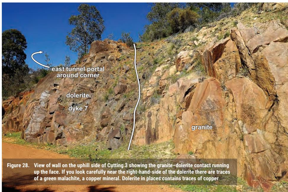
Figure 28. View of wall on the uphill side of Cutting 3 showing the granite–dolerite contact running up the face. If you look carefully near the right-hand-side of the dolerite there are traces of a green malachite, a copper mineral. Dolerite in places contains traces of copper
