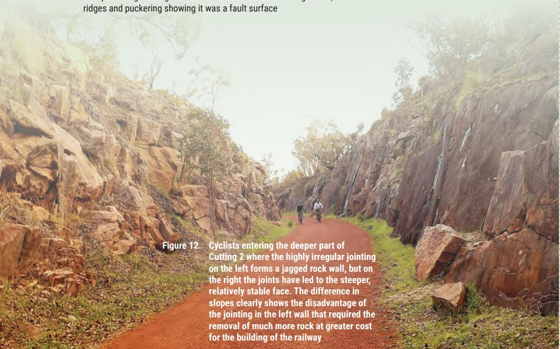
Figure 12. Cyclists entering the deeper part of Cutting 2 where the highly irregular jointing on the left forms a jagged rock wall, but on the right the joints have led to the steeper, relatively stable face. The difference in slopes clearly shows the disadvantage of the jointing in the left wall that required the removal of much more rock at greater cost for the building of the railway
