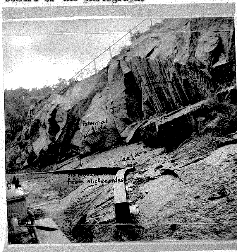
Photo 2: Taken at the rear of the pump house. The joint planes sloping at 22\frac{1}{2}^{\circ} are covered with water from the joint. The 75^{\circ} overhang and a small block in a position of potential block glide are notable.
