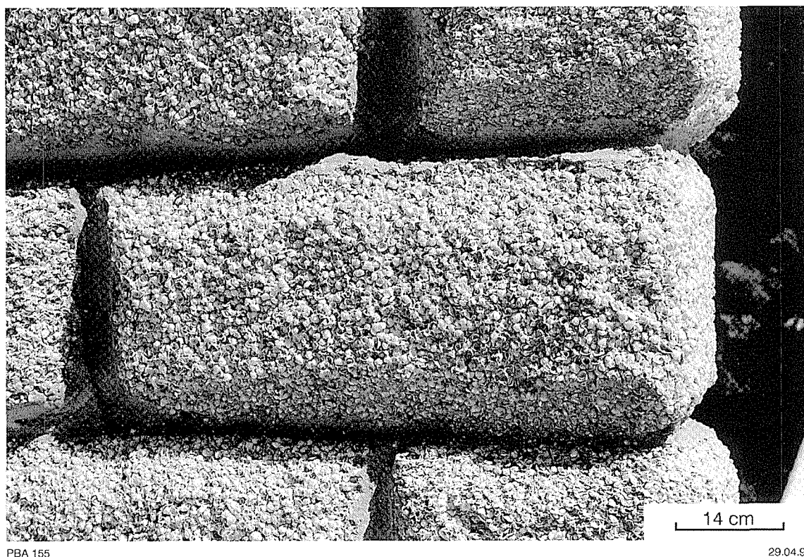
Figure 32. Photograph of coquinite blocks used in the construction and repair of historic buildings in Denham (after Townsend, 1996)
