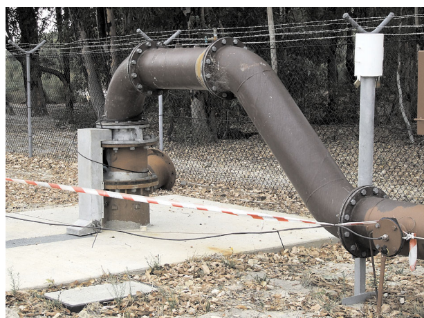
Figure 39. An abstraction bore for Perth's water supply
