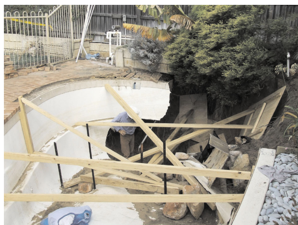
Figure 31. Damage to pool caused by ground collapse
