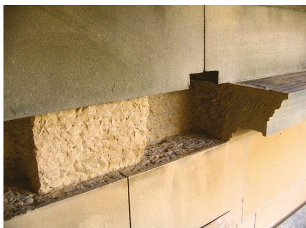
Figure 82. Replacement of weathered sandstone corbel blocks. Sydney Hospital stone restoration project
