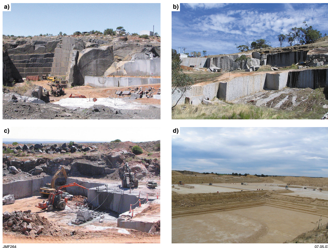
Figure 32. Four basic quarry types: a) near-vertical, quarry cut into the side of a steep hill (Black Hill norite, South Australia); b) benched quarry situated on a moderately sloping hillside (York granite, Western Australia); c) quarry situated close to ground level (Black Hill norite, South Australia); d) below ground level quarry (calcarenite, Moore River, Western Australia)
