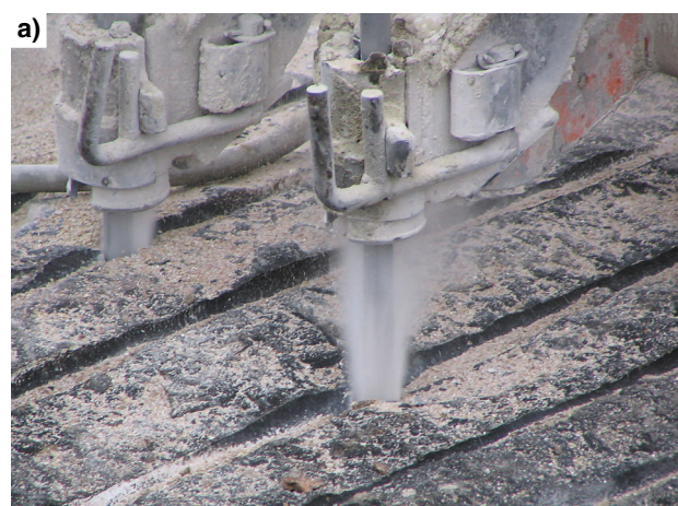
Figure 37. In-line block drilling: a) simultaneous drilling of two holes spaced about 260 mm apart. The next pair of holes drilled will overlap resulting in an in-line spacing of 130 mm; b) a 30 mm-diameter tungsten carbide-tipped button bit capable of rapid drilling in hard rock
