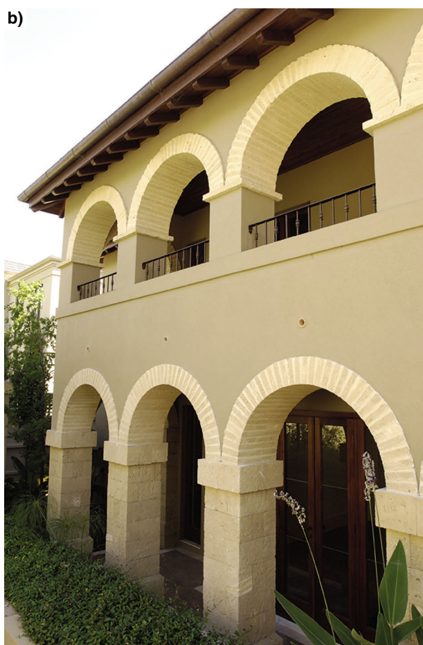
Figure 147. Tamala Limestone from Moore River: a) a six metre-high wall of massive, pale brown, crossbedded calcarenite in the Moore River block quarry; b) Moore River limestone bricks and blocks used in archways and as column cladding in a contemporary Italian-style villa (photo (b) courtesy Limestone Resources Australia, © Discovering Stone, 2006)
