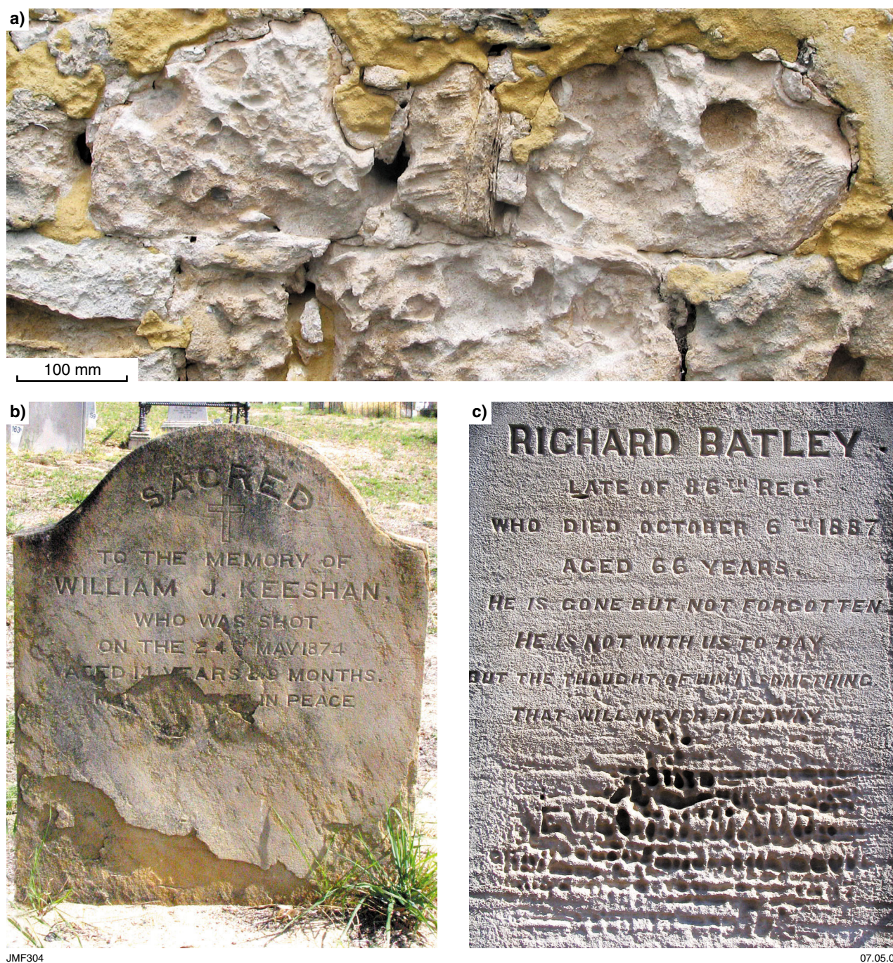
Figure 79. Rain and water weathering effects in limestone and sandstone: a) karstified surface of Tamala Limestone blocks, (Fremantle, c. 1851); b) case-hardened headstone breached by water weathering allowing softer, sandstone matrix to partially collapse; c) honeycomb weathering in sandstone headstone (images (b) and (c) Pioneers Cemetery, East Perth)
